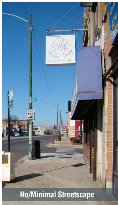
North Avenue Existing Conditions: Oak Park Ave. to Austin Blvd.
