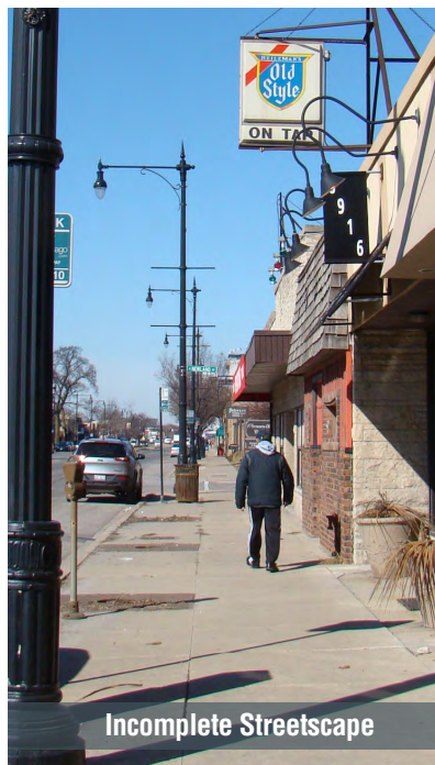
North Avenue Existing Conditions: Harlem Ave. to Oak Park Ave.
