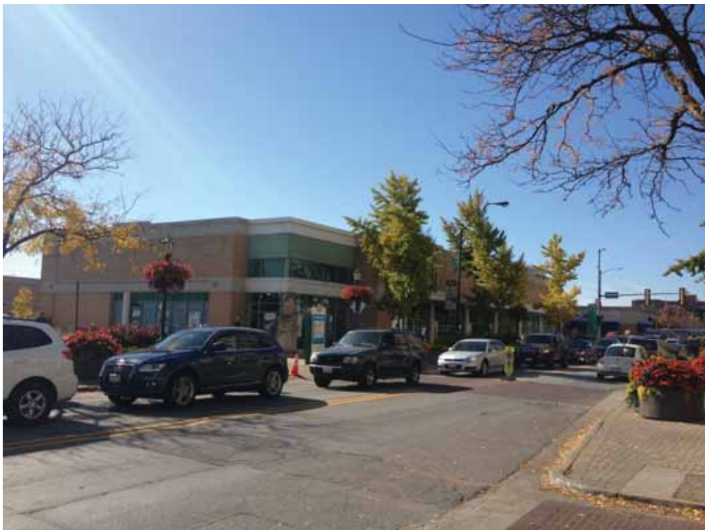
02-LAKE STREET - VIEW TO SOUTHWEST
