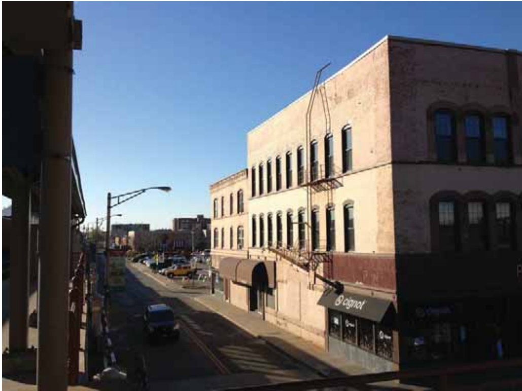
07-NORTH BLVD - VIEW TO WEST AT MARION STREET
