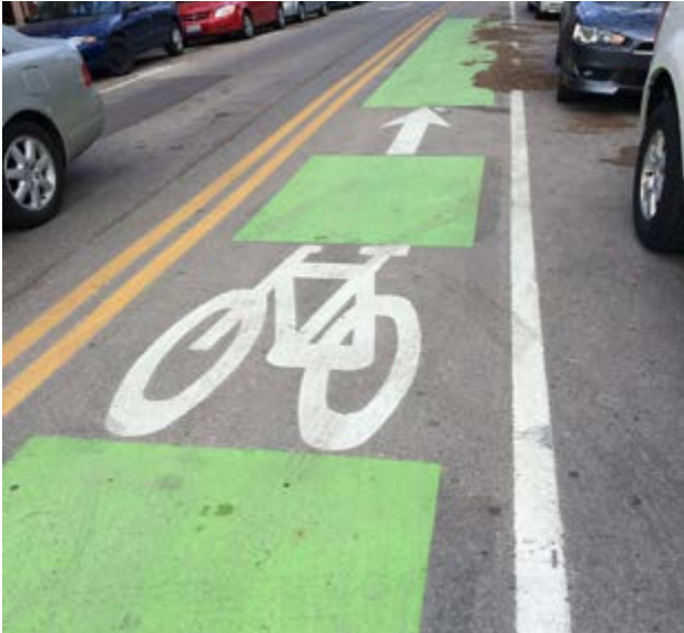
GREEN PAINT May be used near intersections to increase visibility of the contraflow bike lane.
