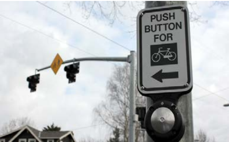
PUSH BUTTONS Enable cyclists to trigger signals, but requires them to dismount. Photo credit: NACTO
