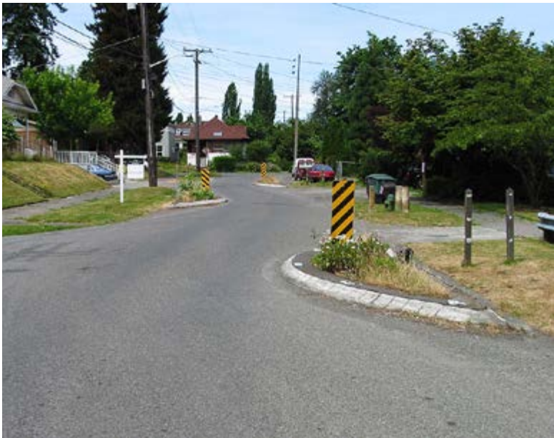
CHICANES calm traffic through horizontal deflection. Photo credit: wikimedia.org
