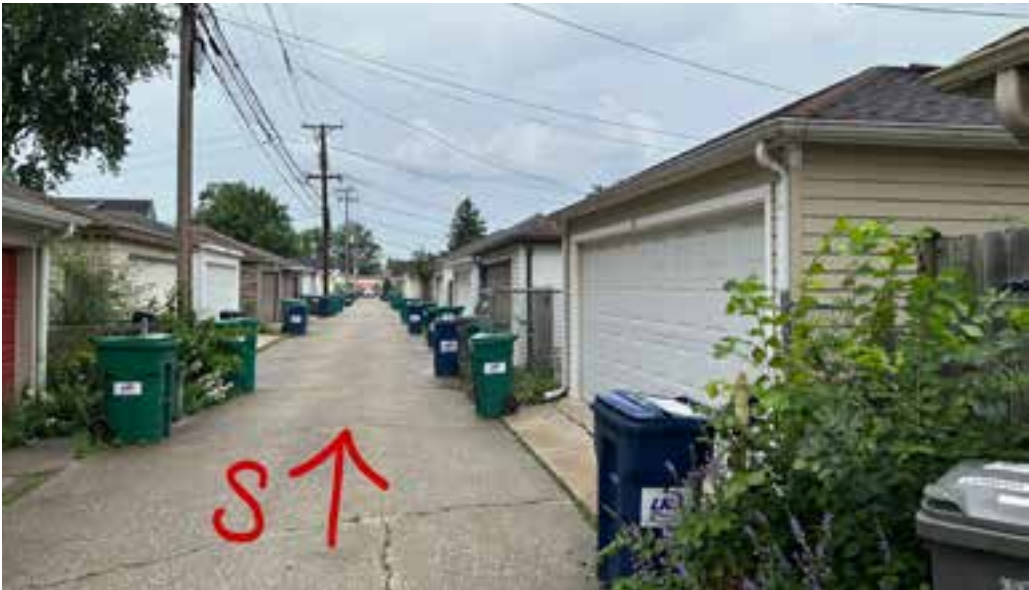
Photo 10. View of Garage of 1152 S. Cuyler Ave, the property South of the existing 1150 S. Cuyler garage
