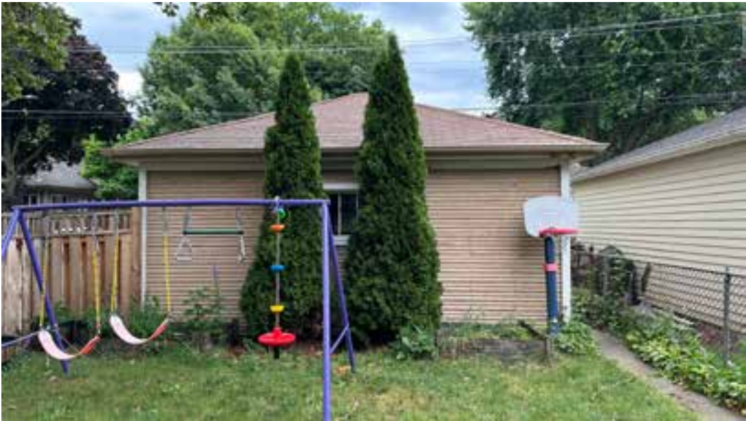
Photo 2. West Side of Garage at 1150 S. Cuyler, facing East.
