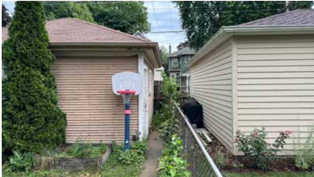
Photo 3. South Side of Garage at 1150 S. Cuyler between 1152 S. Cuyler's Garage. Facing East.
