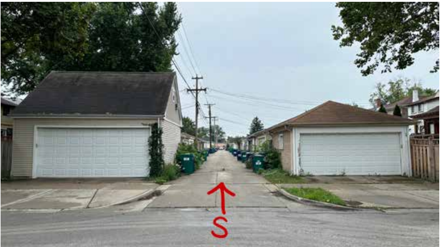
Photo 8. View of Alley between existing Garage (1150 S.Cuyler) and neighboring garage (1151 S. Highland Ave).
