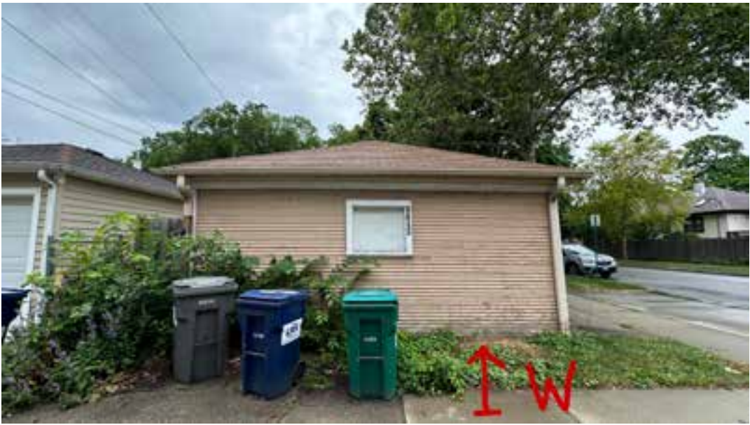
Photo 1. East Side of Garage at 1150 S. Cuyler
