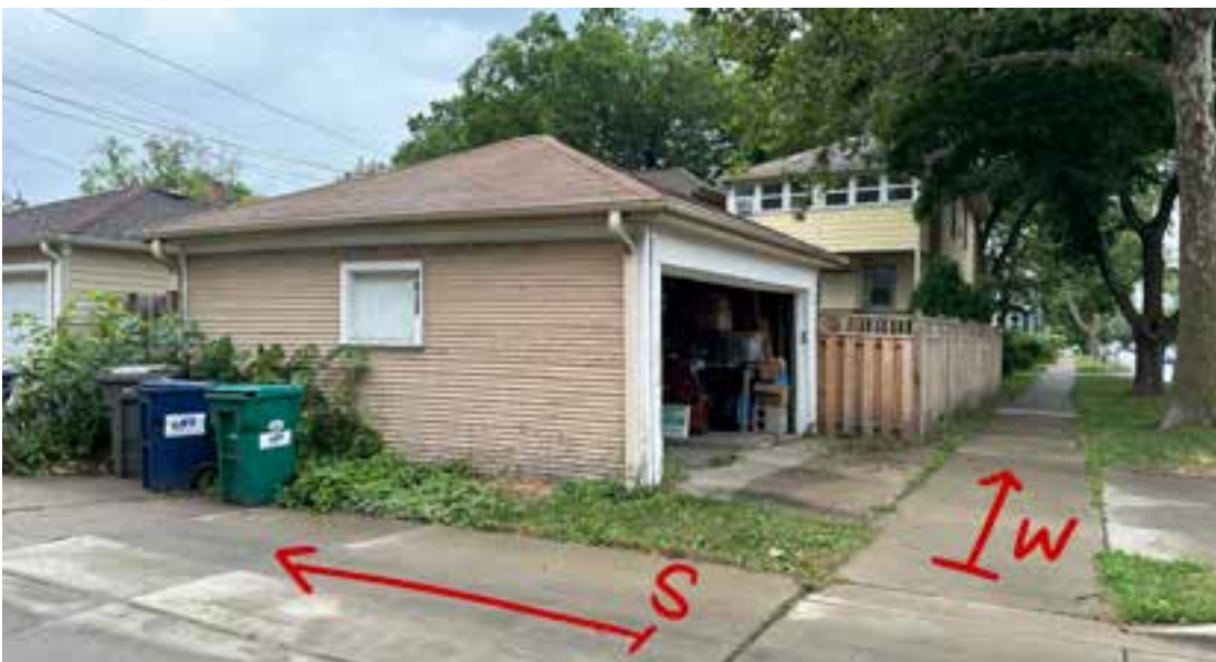
Photo 6. View of Existing Garage from alley at 1150 S. Cuyler
