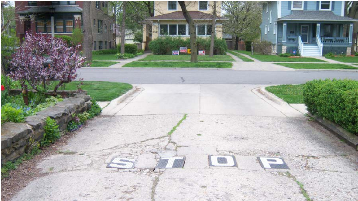
Oak Park alley stop sign (Village photo)
