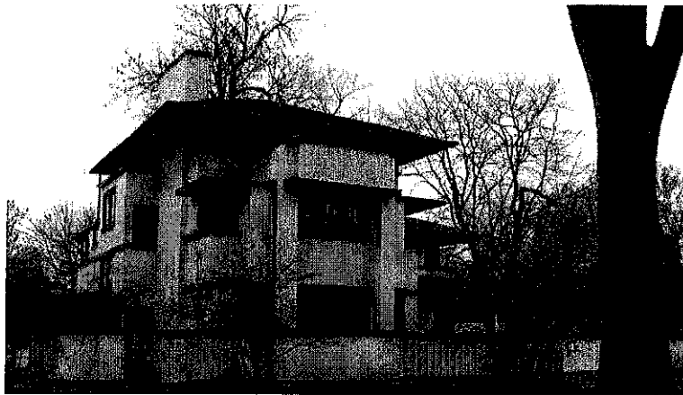
Figure 30: William E. Martin House, 636 N. East Avenue.
