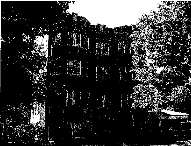
Figure 88: Apartments built ca. 1920 at 1035-1037 Superior Street.
