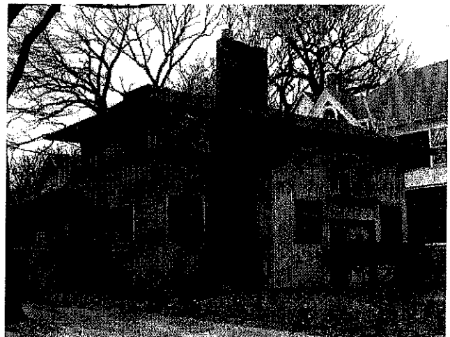
Figure 48: H. Benton Howard House (1904) 911 Chicago Avenue.
