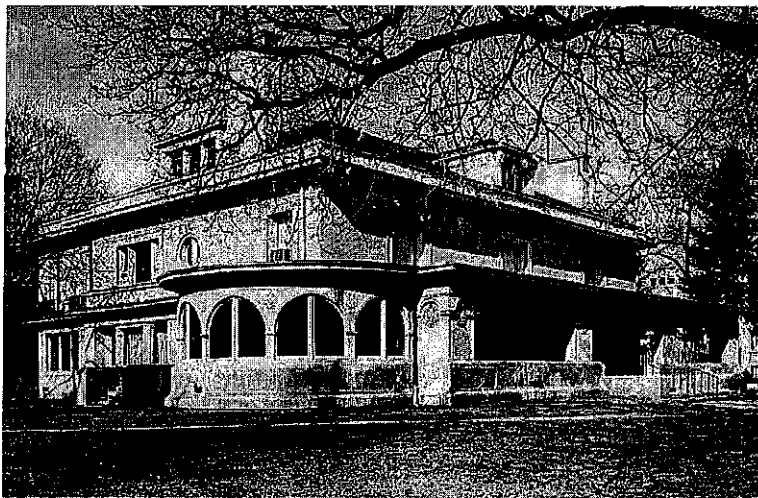
Figure 64: John Farson House, (1897) 217 Home Avenue.
