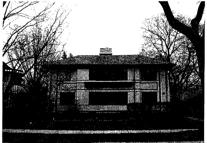
Figure 56: E.P. Ward House (1915), 724 Linden Avenue.
