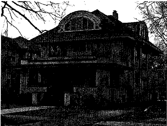
Figure 51: Louis H. Brink House (1909), 533 N. Grove Avenue.
