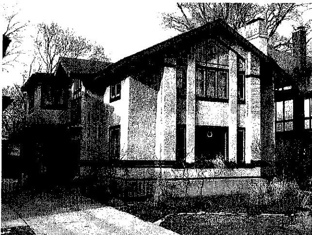
Figure 59: Harold H. Rockwell House (1910), 629 N. Oak Park Avenue.
