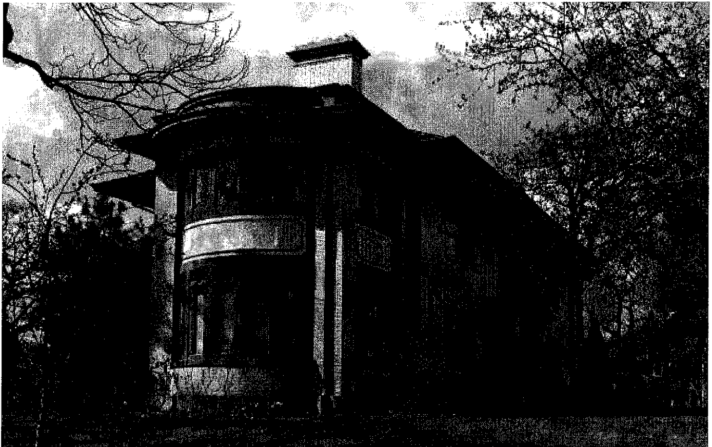
Figure 66: James Hall Taylor House (1912), 405 N. Euclid Avenue.
