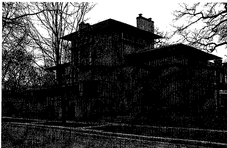
Figure 28: William G. Fricke House, 540 N. Fair Oaks Avenue.
