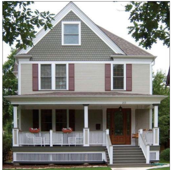
The original porch was missing and replaced with a compatible style, including scale and setback.
