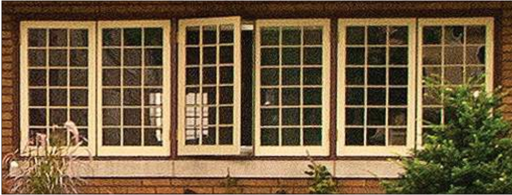
This band of three paired 18-light, wood casement windows have true divided lite muntins. The windows provide interior illumination and allow for ventilation.
