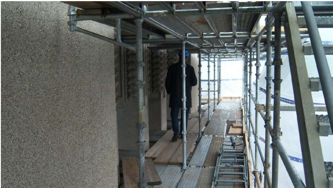
Unity Temple restoration project 2015 (Village photo)
