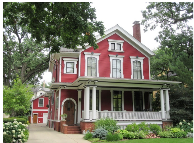
Oak Park Landmark, the John Schmidt House, was built ca. 1872 and renovated by prominent local architect E.E. Roberts in 1908.
