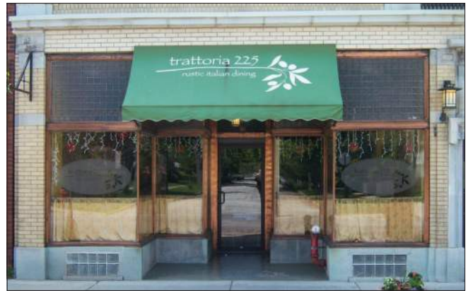
These transom windows are made of Luxfer prism glass, which was invented in 1896 and designed to refract and spread additional light towards the back of the store.
