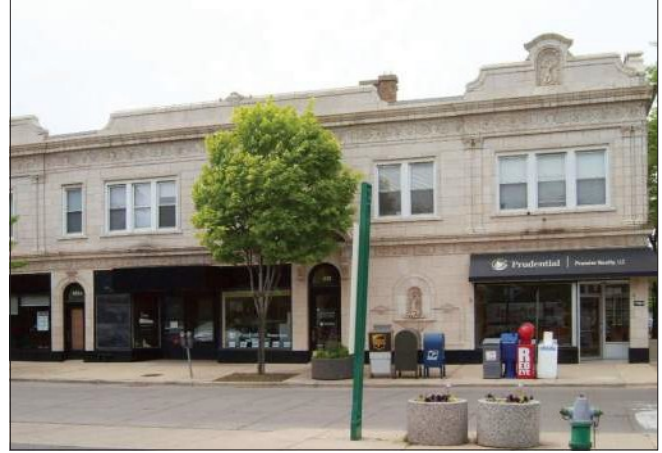
The storefront cornice visually separates the storefront from the upper building levels.
