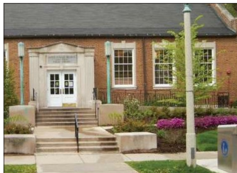
This library has an accessible ramp that both maintains the original entrance steps and allows all patrons to utilize the main entrance door of the building.
