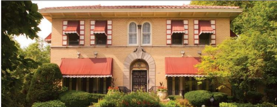
Many of Oak Park's apartment buildings are brick with limestone trim. This is a less-common, single-family residential example.
