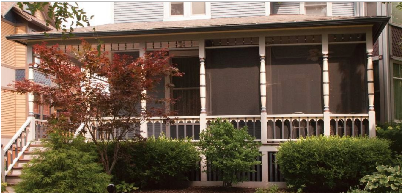
The right side of this porch has been enclosed with insect screens. The screens are installed behind the columns and the balustrade and the supporting structure is not visible from the public right of way.
