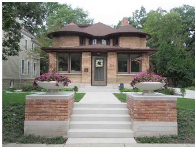
Site elements such as sidewalks, stairs, posts, urns, and walls may be key elements in defining a building's context and character.
