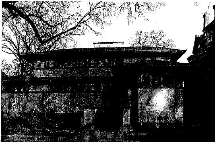
Figure 25: Frank W. Thomas House at 210 Forest Avenue.
