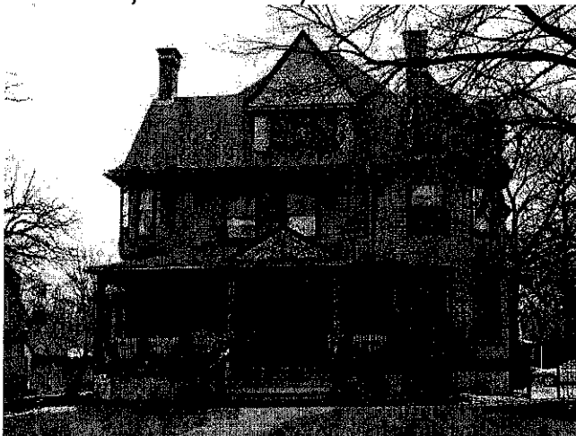
Figure 8: John Rankin House at 245 N. Kenilworth Avenue (1891) designed by Patton & Fisher.
