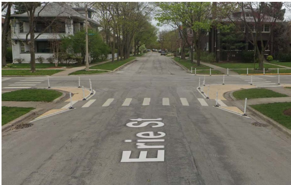
Figure 5. Paint and Post Curb Extension Example
