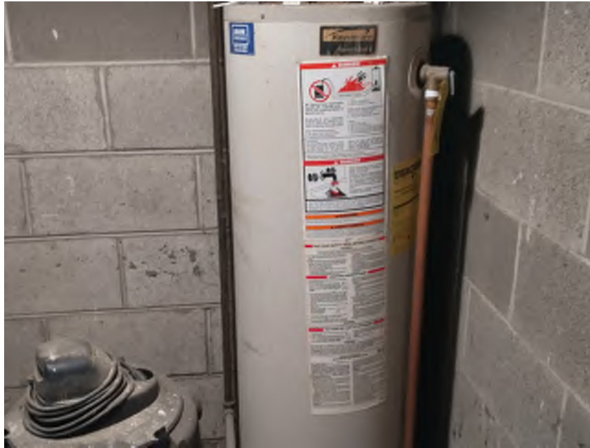
Photograph No. 9 View of the interior - furnace room
