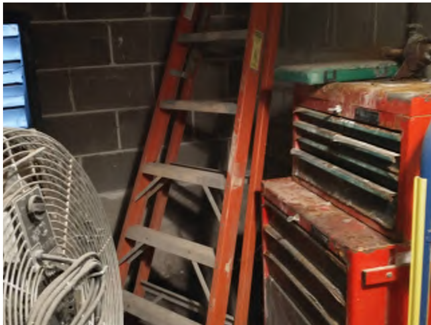
Photograph No. 10 View of the interior - furnace room
