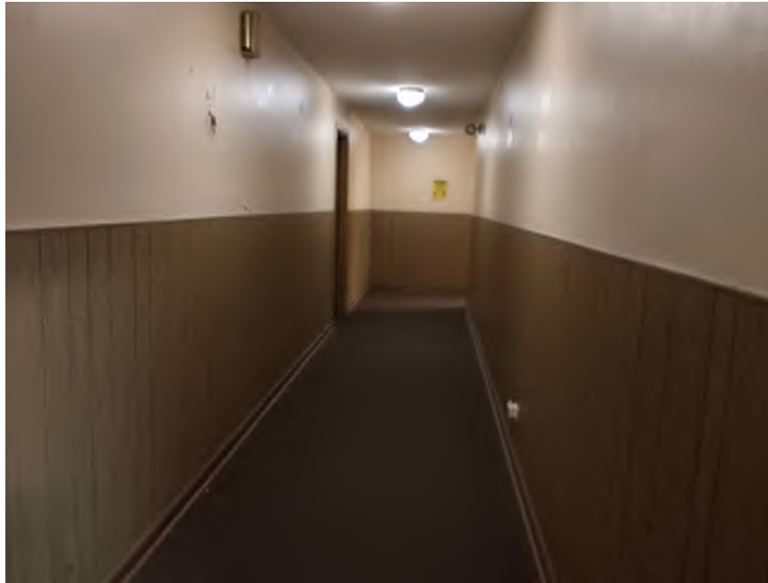
Photograph No. 7 View of the interior - first floor hallway
