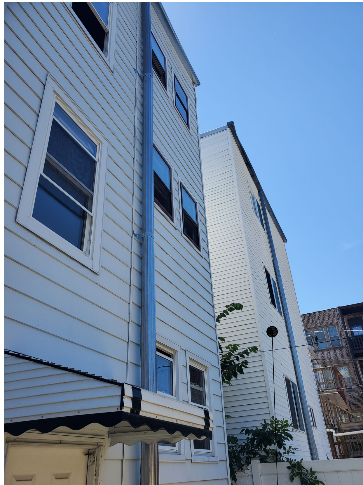
112 S. AUSTIN BLVD, OAK PARK, IL - BUILDING REAR
