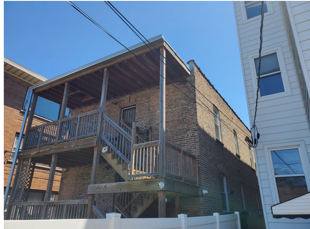
108 S. AUSTIN BLVD, OAK PARK, IL - BUILDING REAR
